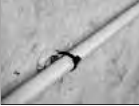
Flexible or rigid cable conduits with cable ties
