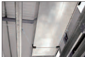
Square Air Ducts
