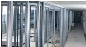
Drywall tracks to concrete and steel
