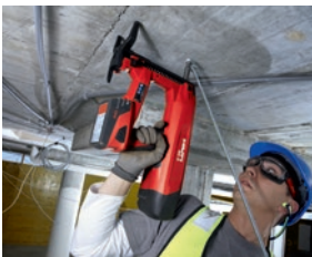
Threaded rod attachments to concrete
