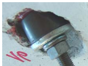
Fig. 11: anchor head in concrete
