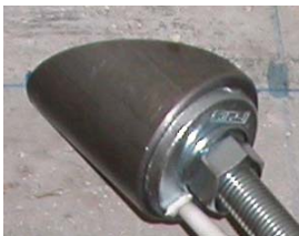
Fig. 10: anchor head external
