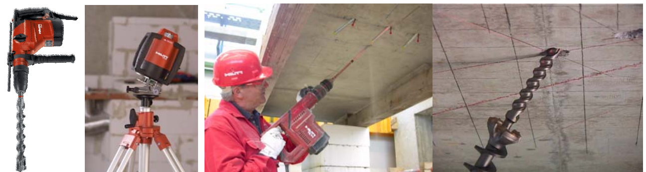
Fig. 13: drilling of the holes
