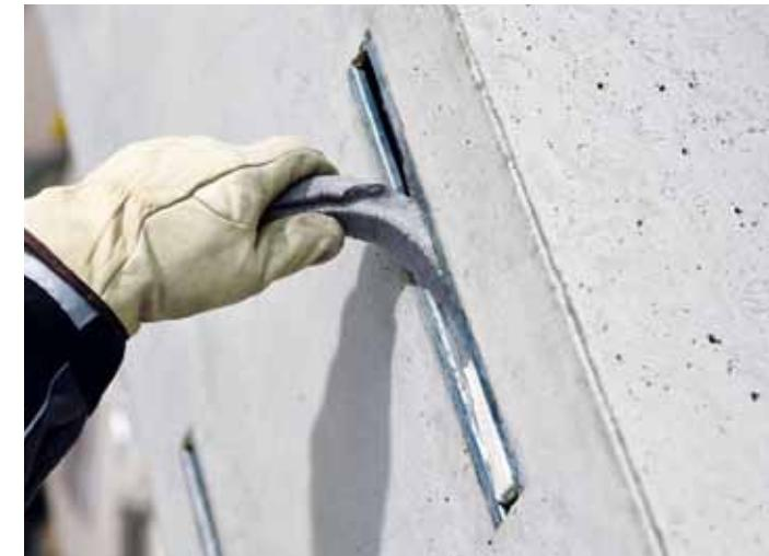
The classic anchor channel cross section has been optimized with the aid of advanced computer simulation and through intensive testing. The resulting innovative V-form takes up high loads and allows small edge distances at edge zones where shear loads occur.
