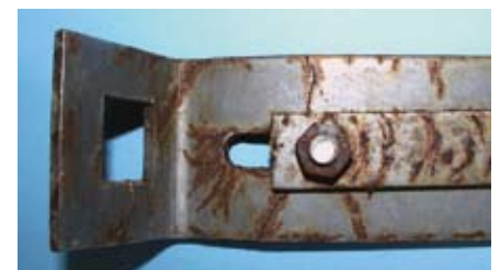
This shows SCC of a retaining strap made of the material 1.4301 (A2, 304) after approx. 4 years of use in an indoor swimming pool (CH).
