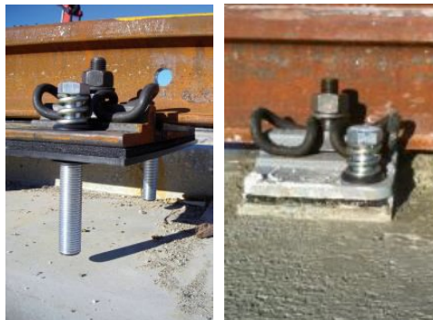
Clipped components before concrete pouring
