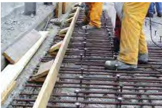
Slab strengthening
